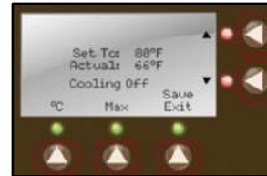
Adjust Temp/ Cooling On
